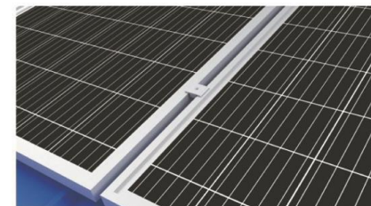
6 安装组件, 用侧压块将组件与导轨固定。 Solar panel mounting, fix the panel on rail with end clamp.
