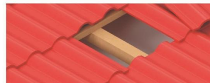
1 根据方案图，将需要取下的瓦片取下。 According to the scheme drawing, remove the tile.
